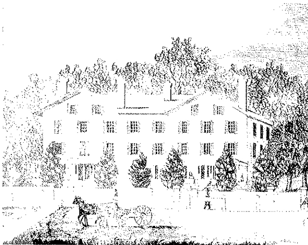
FRONT VIEW OF THE ORIGINAL BUILDING
